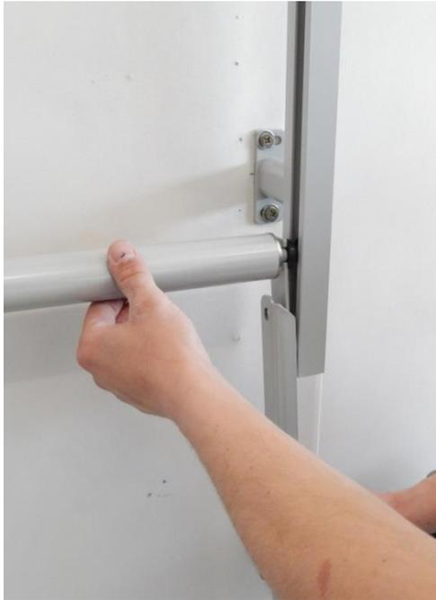
1. Insert the intermediate bar into the arm cutouts and insert the whole into the guide rails.
