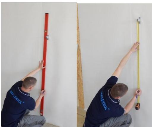
4. Measure and mark places for installation of the remaining brackets.
