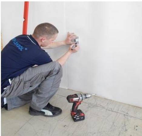
1. Designate spots in the axis of installation of side guide brackets to the base. Put the bracket on the base and mark places for installation holes.
