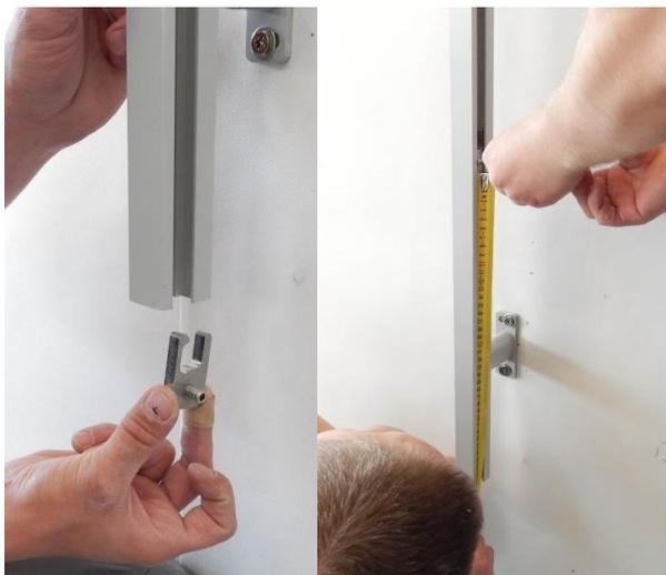
2. Insert the arm lock into the guide rails, And then lock it at the previously measured height.
