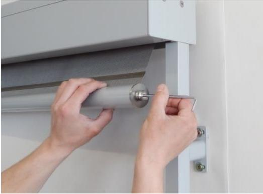
2. Connect the drive to power supply and unroll the fabric, then unscrew the bolts in the bottom bar that are used to assemble the movable part of the arm.
